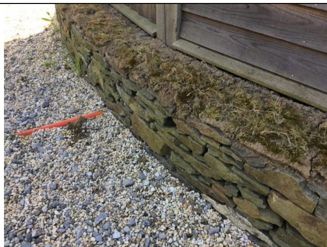
Photograph 11: Stone wall at the base of Building 2
