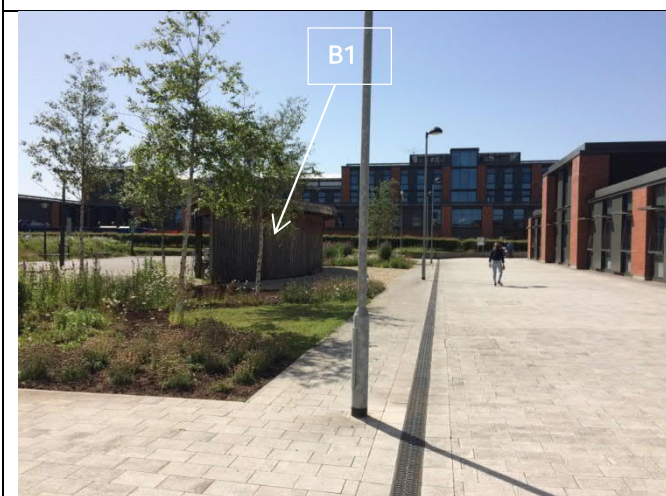
Photograph 5: Native species planting and scattered trees. With surrounding areas of hardstanding and Building 1 (cycle store) with green roof.
